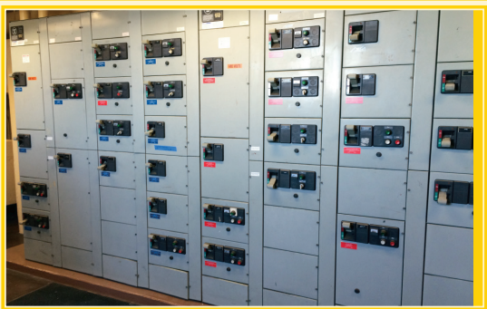
WTP Switch Gear – Showing red/blue tags identifying the power grid feeding the panels
