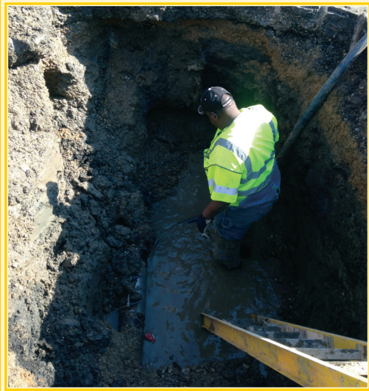
Lewis Ave Water Main Leak Repair
